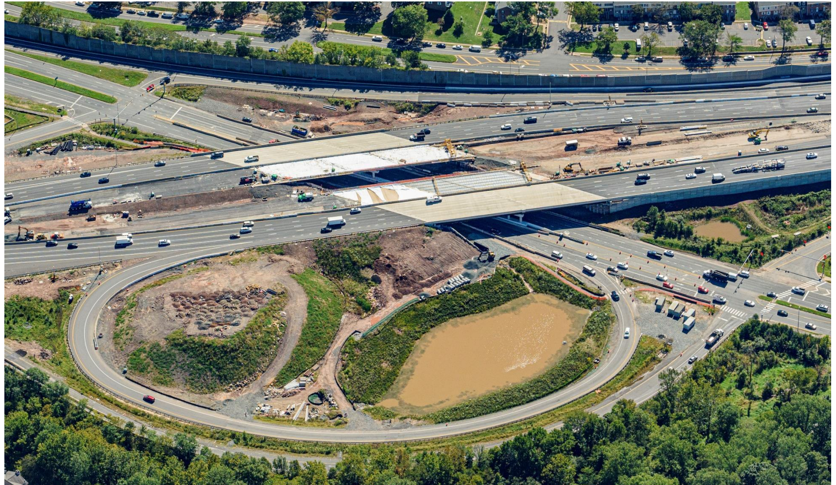
September 2021, Route 29 Interchange
