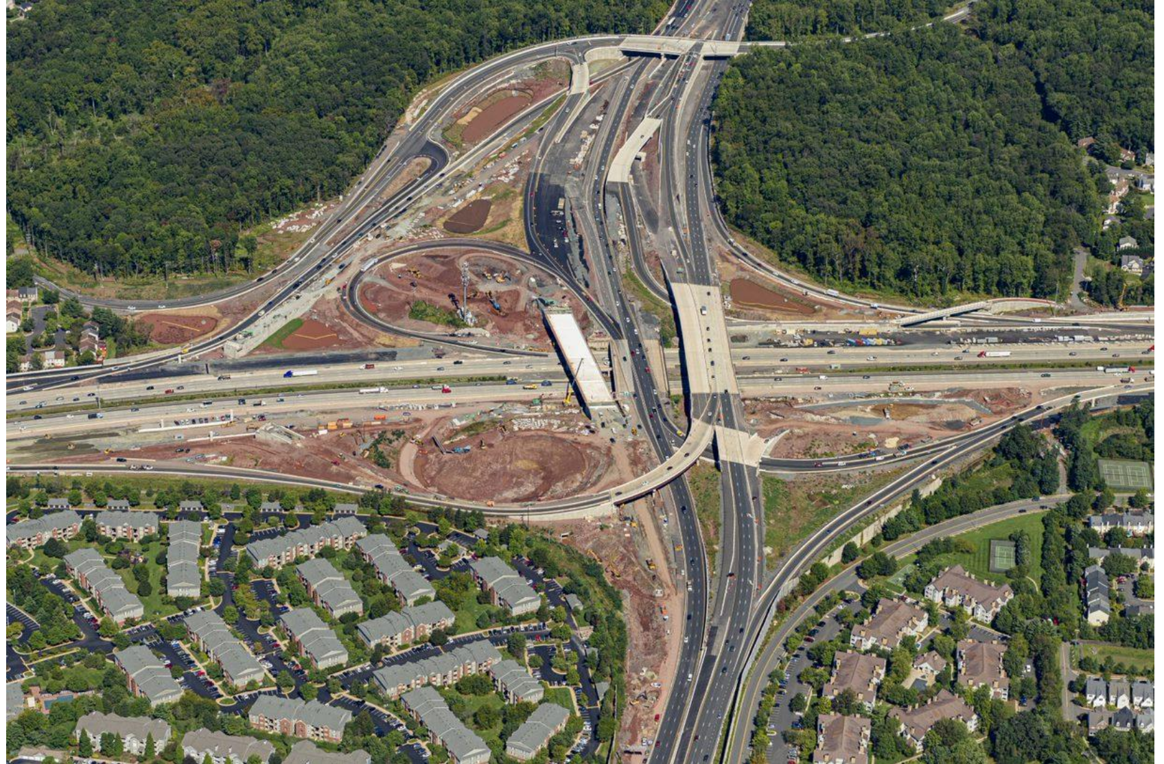
September 2021, Route 28 Interchange
