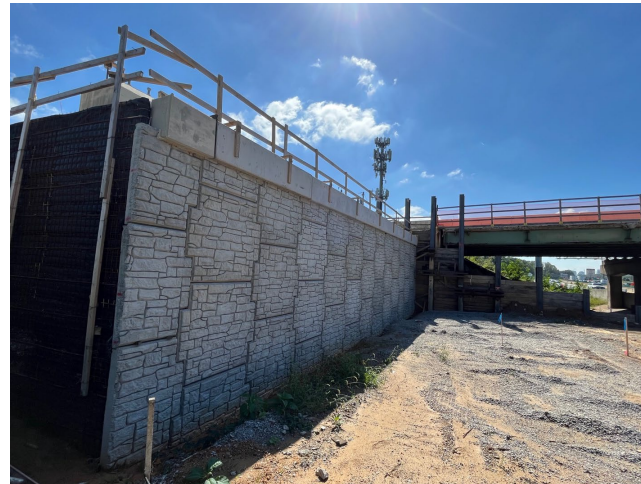
Recently-completed eastern abutment for new Georgetown Pike bridge.
