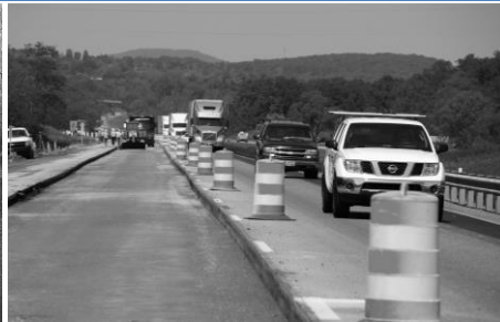
I-81 Pavement Project
