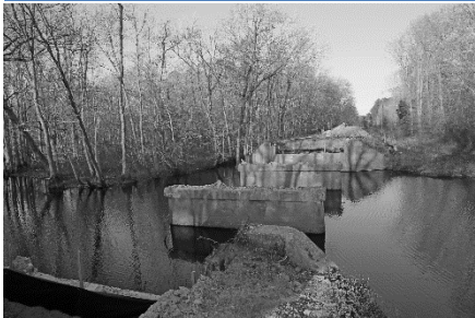
Carson Road (Rte 703) Bridge Replacement
